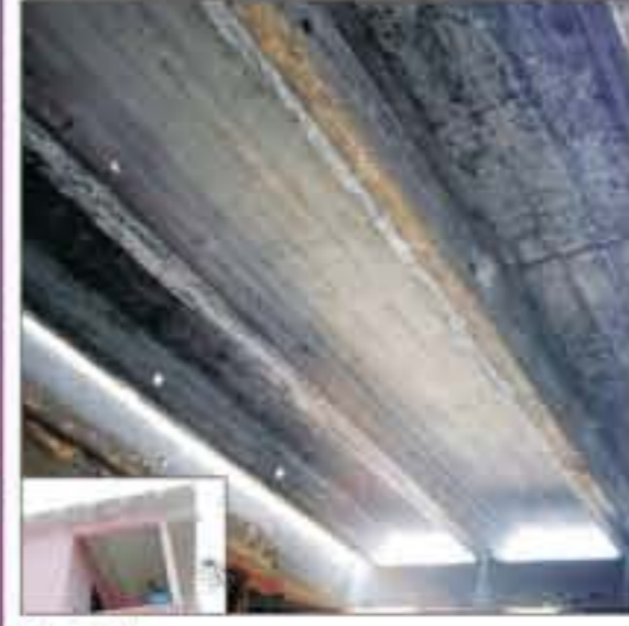
Losa canal CTDMC, Cuba
