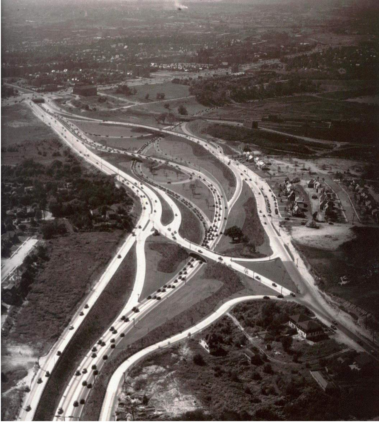
Union Turnpike, Interboro Parkway e Queens Boulevard. 1937
